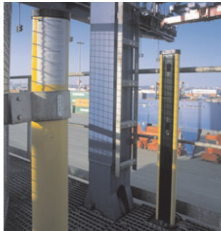
Port: Access protection on a container bridge
