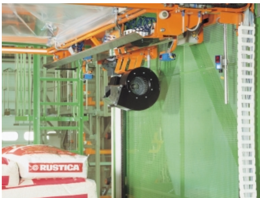
► WT 30 photoelectric proximity switches detecting the location of pallets to control the path of the shrink-wraper.
